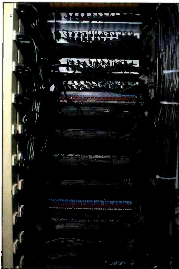
A rear view of the ADC audio patchbay setup (left) and the Symetrix auto-levelers (right).
